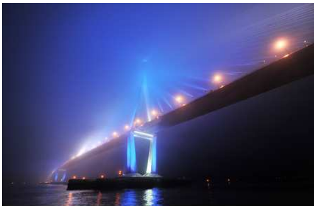
Incheon Bridge is lit up after completing the second round of installation of lights, last week.
